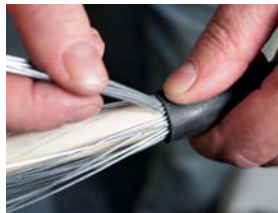
STEP 3: REMOVE OUTER SHEATH
