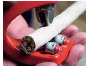
STEP 5: LONGITUDINAL CUT AND REMOVAL OF SECONDARY SHEATH
