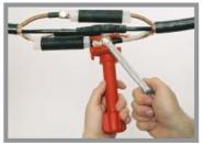
Jointing of the conductor is performed with a screw through connector. Tighten the screw with a socket wrench until it breaks at the groove.
