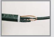
The outer insulation is then installed, and the core is drawn out in the same way as in the previous item and shrinks the hose immediately.
