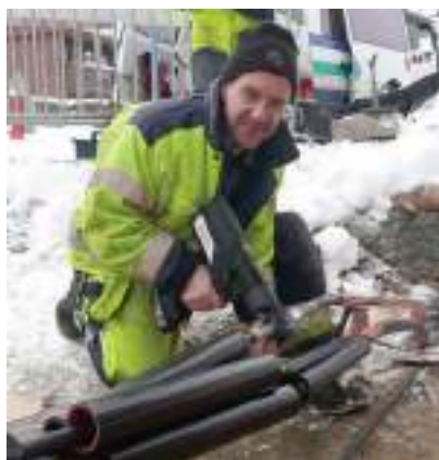
Crimping with Elpress crimp tool PVL1300.
