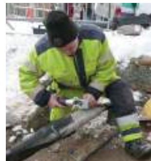
Crimping with Elpress crimp tool PVL611.
