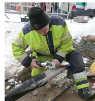
Crimping with Elpress crimp tool PVL611.
