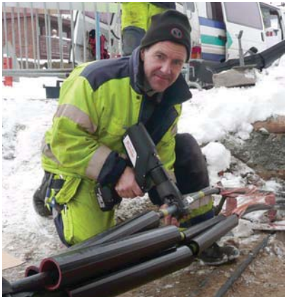
Crimping with Elpress crimp tool PVL1300.
