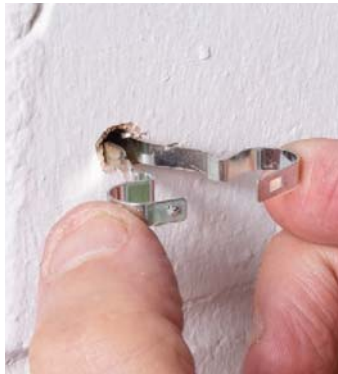
Drill pilot hole & select appropriate size of Stag Clip
