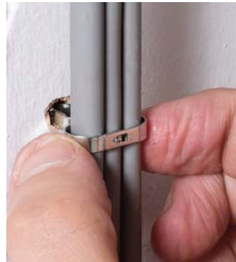
Insert cable(s) before squeezing the smooth head
