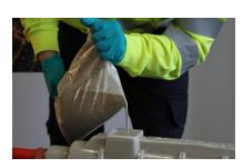
8. Finally cut one corner and pour the contents into the joint shell.
