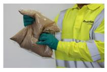
7. Tumble mix and knead the bag for up to two minutes, to ensure that there are no lumps in the bag.
