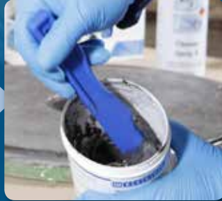
Mix resin and hardener thoroughly and bubble-free
