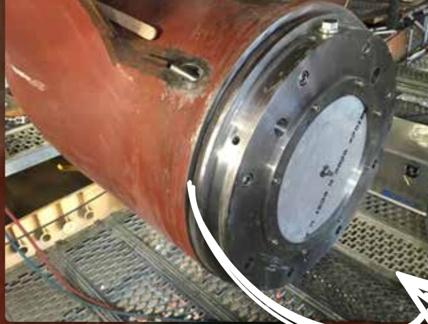
Repair of a shaft seal ring on a ship propulsion system Urethane 80 Putty
