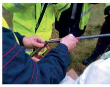
3. The earth line is locked to the hardened steel tip with the leading rod.
