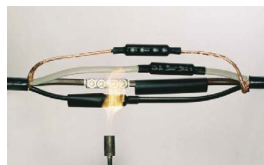
Shrinkage of the insulation is achieved by using heat.
