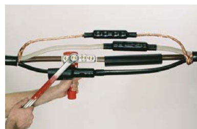
Conductors are spliced using shearbolt connectors Tighten the screw using a socket wrench, until it shears in the cut-off groove.
