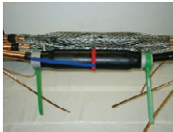
Joint body in position
