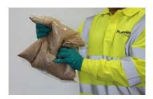
7. Tumble mix and knead the bag for up to two minutes, to ensure that there are no lumps in the bag.
