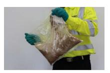
6. Before mixing rotate and shake at the corners to free the powder.
