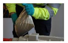
8. Finally cut one corner and pour the contents into the joint shell.
