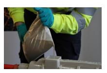
8. Finally cut one corner and pour the contents into the joint shell.
