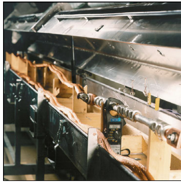
Test of terminals.
