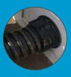
5 Hand-tighten the AQUA-Nut to the outside of the chamber/catchpit wall.
