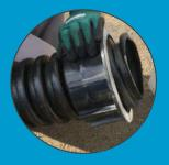
From inside the chamber/catchpit, screw the AQUA-Mouth into EFLEX Round.
