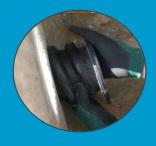
3 Insert EFLEX into the chamber/catchpit wall.
