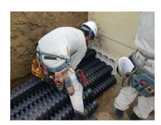
When the EFLEX Square ducts meet at the centre point of the section, the length can be adjusted and the AQUA Square accessory is used to complete the installation (see AQUA Square connection procedure on page 9).
