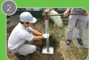
2 Drive column into the base plate
