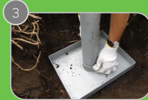
3 Secure column to the base plate with included nut and bolt
