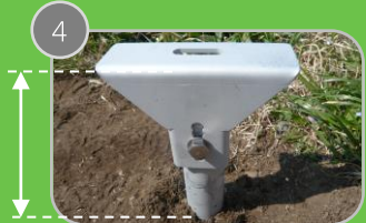
4 Backfill and attach the steel pedestal
