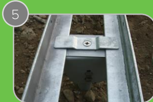
5 Attach the steel tray to the pedestal using included fixture
