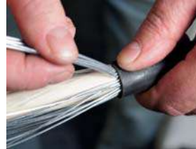
STEP 3: REMOVE OUTER SHEATH
