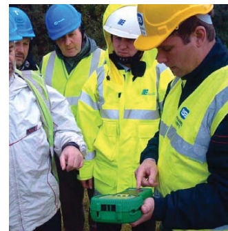
Measuring earthing resistance of the earth connection
