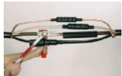
Conductors are spliced using shearbolt connectors Tighten the screw using a socket wrench, until it shears in the cut-off groove.
