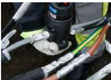
Indent crimping of Elpress through connector using crimp head V250.
