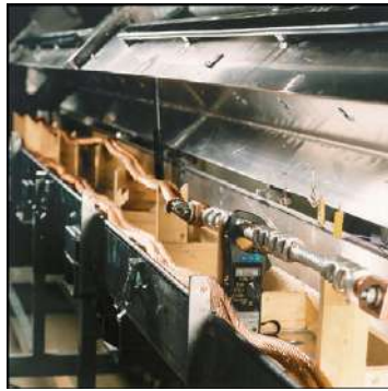
Test of terminals.
