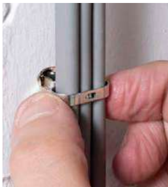
Insert cable(s) before squeezing the smooth head
