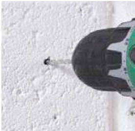
Drill a 5mm pilot hole
