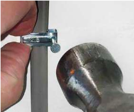
For 2.5mm 2 flat twin & earth cable
