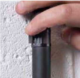
Secure cable with locking tab
