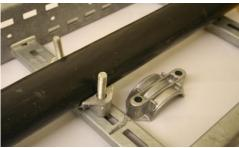
Locate the other half of the cable clamp. Secure with 2 fastening nuts and washers (not supplied) and tighten.
