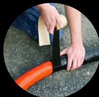
Repair for substantial cable jacket repairs
