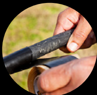
Repairing minor scratches on cable jackets
